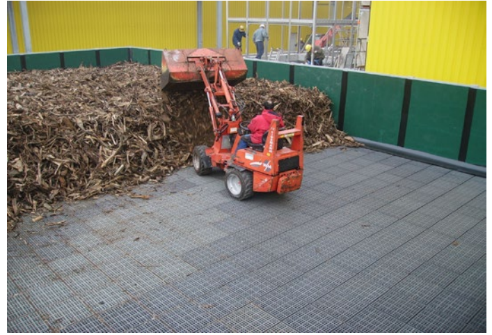
2-ton trucks can drive on it immediately ...
